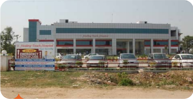
Healing Touch Hospital Ambala Before ● ₹ 5 Mn / month (April-2020) At the time of acquisition
